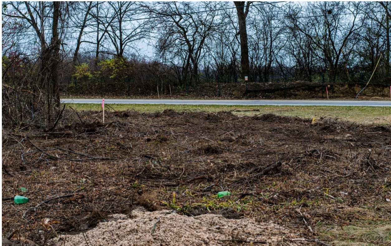
Figure 4 Pre-construction. Survey workers placed right-of-way markers around the proposed project site to mark where the future roundabout will be.
