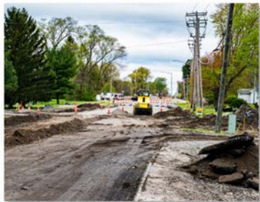
3 Roadway Improvement Projects
