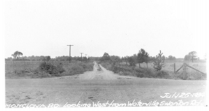
Monclova Road at Waterville Swanton Road Looking West - 7-25-1934
