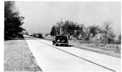
Newly Finished McCord Road-Springfield Twp. WPA Concrete Paving Project c. Mid to Late 1930s
