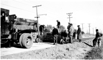
Laying Asphalt-Location Unknown c. 1934
