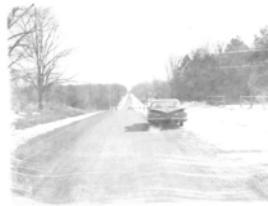
Monclova Road Looking West at Bridge #395 over Swan Creek - 3-2-1962
