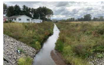
9/27/2022 Post Construction—Zink Heldman Ditch Hybrid Two-Stage Ditch Looking Southeast—Springfield Township
