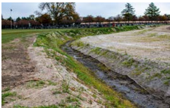
10/22/2022 Post Construction—Van Fleet Ditch Hybrid Two-Stage Ditch Looking East—Monclova Township
