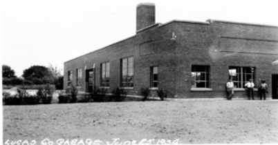
The Nearly Completed LCE Road Maintenance Garage (WPA Project) 6-25-1934
