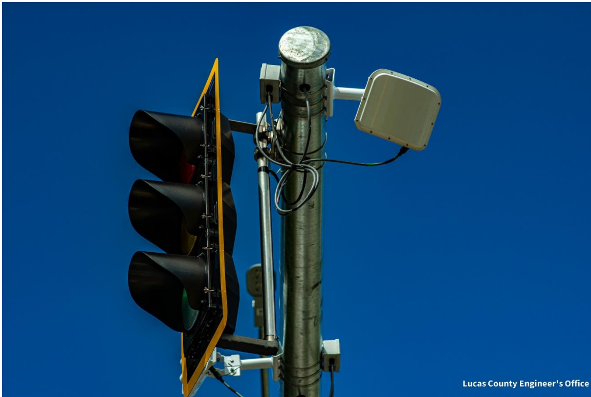
Figure 3 Radar detection devices are attached on the new traffic signals to help detect people on the trail before they even make it to the intersection.
